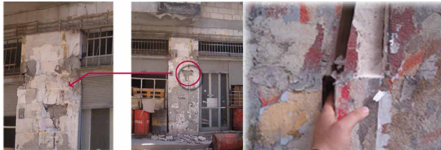
Figure 3. Masonry Building (5 floors), crack patterns in masonry pillars and expulsion of blocks.
