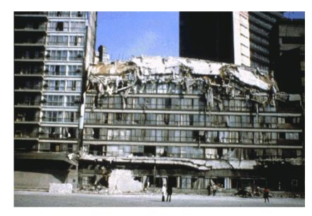
greater damage at 5 to 15 storey buildings despite <u>distance > 350 km</u> from ipocentre
