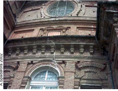
In 1985, concerns over such severe cracking, prompted the decision to undertake monitoring and strengthening works.
