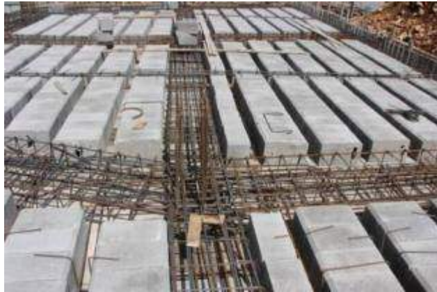
One way ribbed slab system
