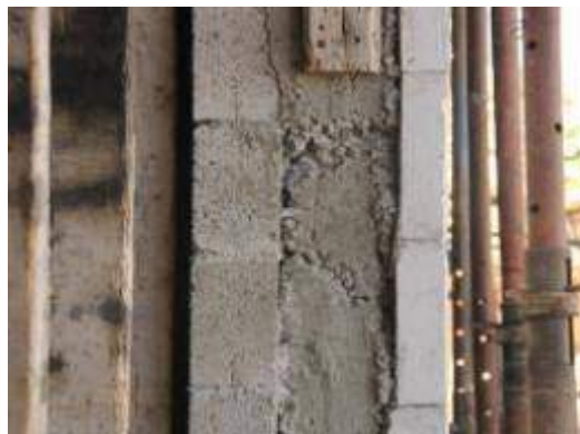
Cross Section of Exterior Masonry Wall
