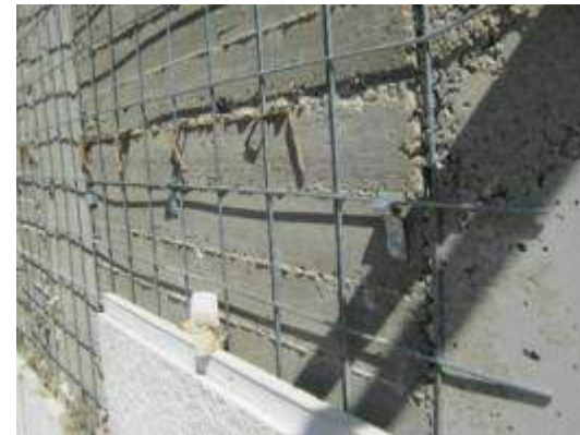
Reinforcement Used to Fasten the Stone Cladding to the Shear Wall
