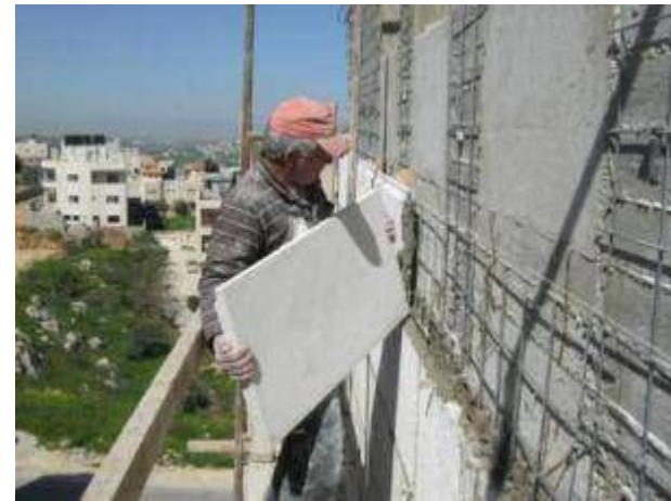
Stone Cladding of Shear Wall Building
