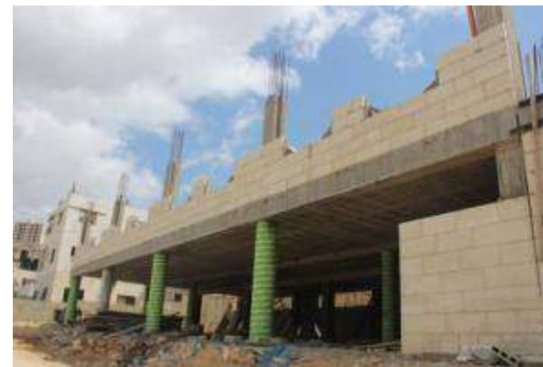
Circular Concrete Columns in an R.C. Frame Building
