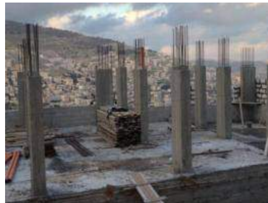
Concrete Columns in an R.C. Frame Building
