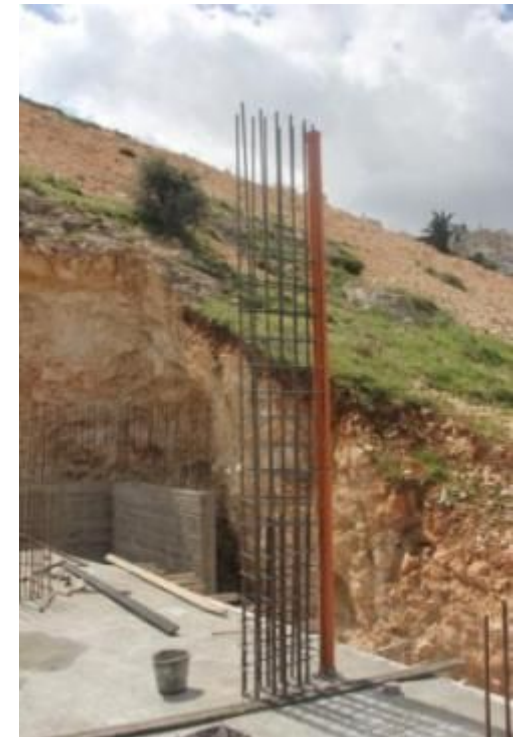
Steel Cage for a Concrete Column in an R.C. Frame Building
